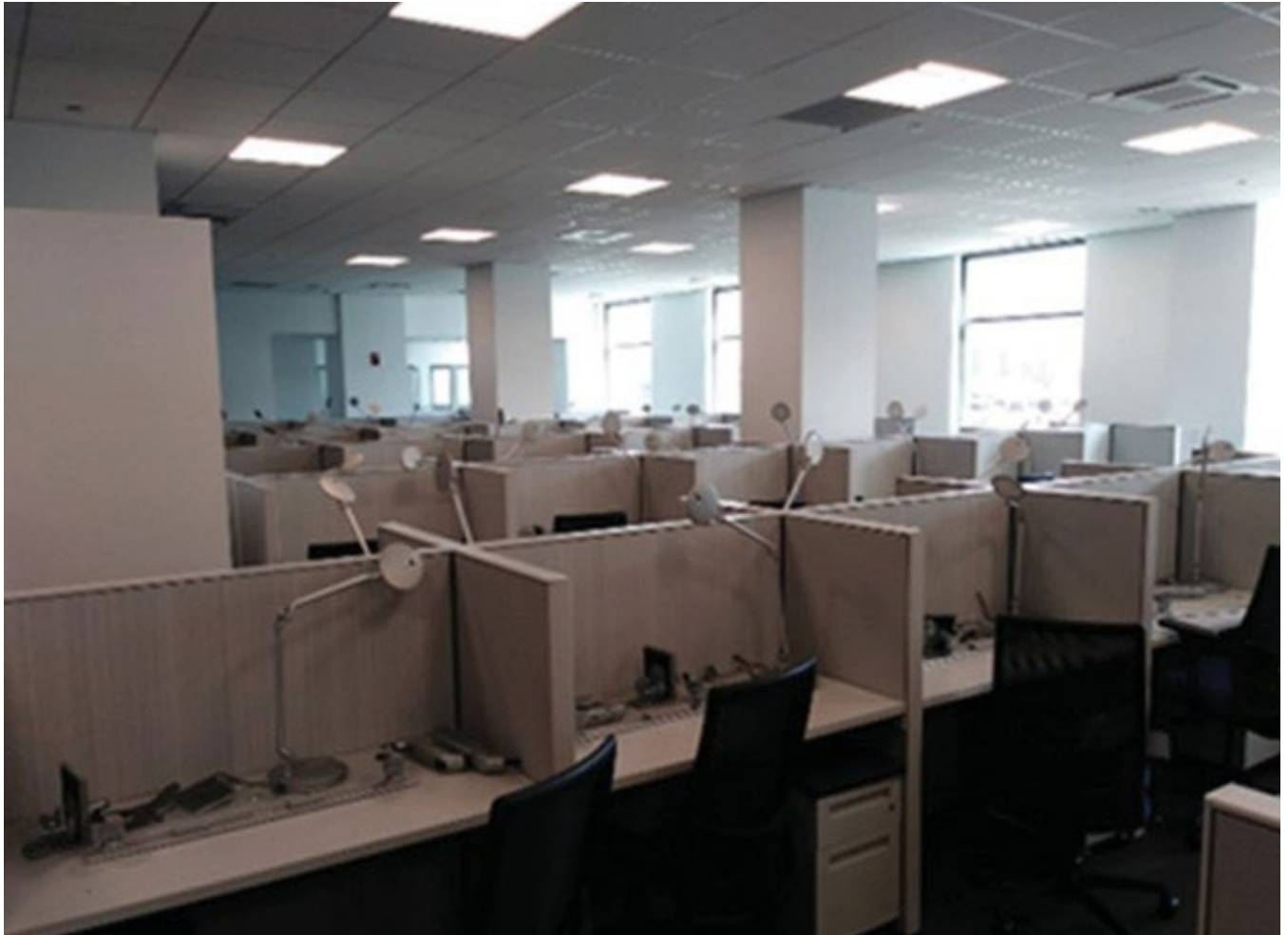
Harrison Square Interior Buildout
