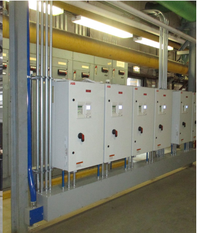
New Cooling Towers at DOC Powerhouse Medicine
