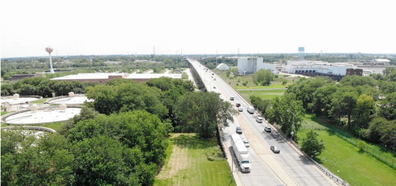
The nearly 1-mile long Central Avenue Bridge spans the Sanitary & Shipping Canal, MWRD Southwest Sewage Treatment Plant, and BNSF and Canadian Pacific Railroads. The bridge's proximity to the I-55 interchange adds complexity for staging the improvements.
