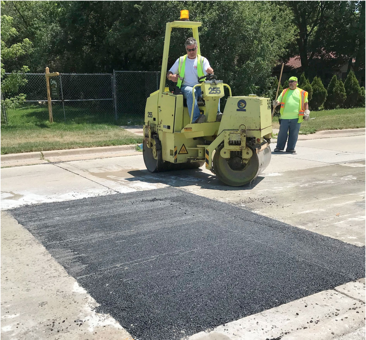
Cook County maintenance crews repair and maintain asphalt and concrete pavement surfaces, ensuring safe and efficient traffic flow on Cook County roadways.
