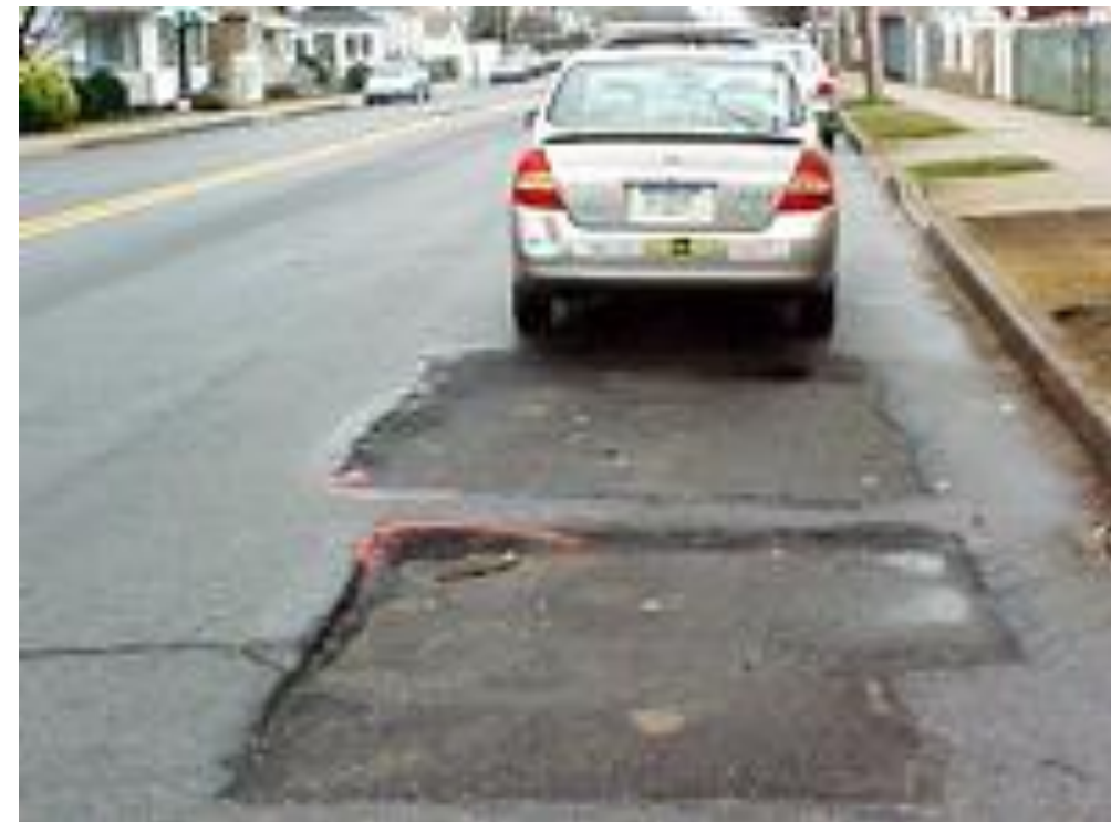
Example of poor patches that need to be addressed
