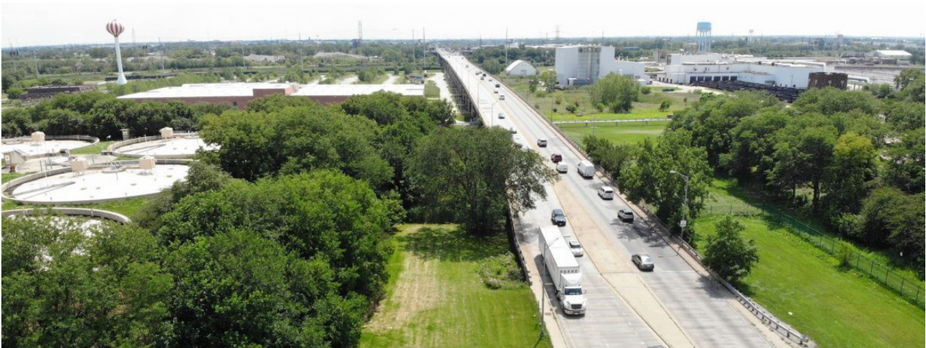
The nearly 1-mile long Central Avenue Bridge spans the Sanitary & Shipping Canal, MWRD Southwest Sewage Treatment Plant, and BNSF and Canadian Pacific Railroads. The bridge's proximity to the I-55 interchange adds complexity for staging the improvements.
