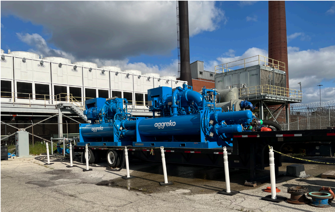
New cooling towers and chillers at DOC powerhouse
