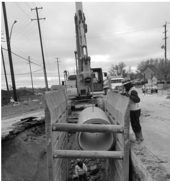
Figure 3. Installation of new storm sewer on the Lake Cook Road project.
