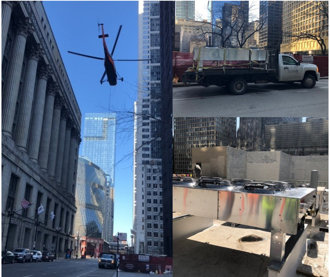
Installation of new rooftop condensing unit on County Building for Bureau of Technology Data Center
