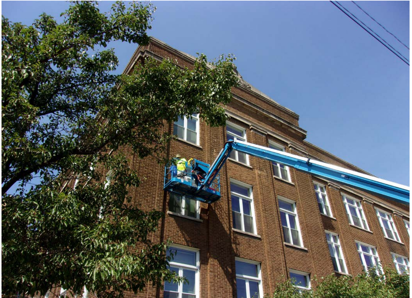
Window Replacement and Re-roofing projects at the South Campus of the Department of Corrections
